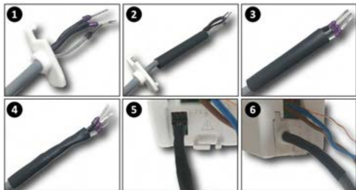
Figure 11. Details for Connecting Modbus Communications Wiring
